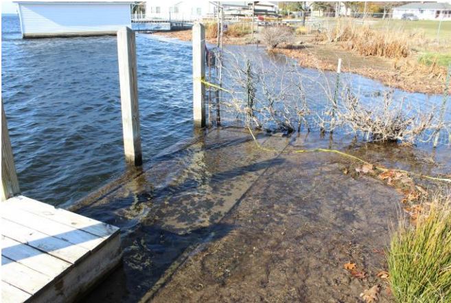
2020 High Water Flooding
